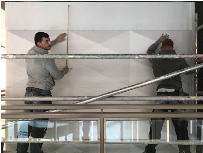
Jason and Jake installing the casts onsite.
